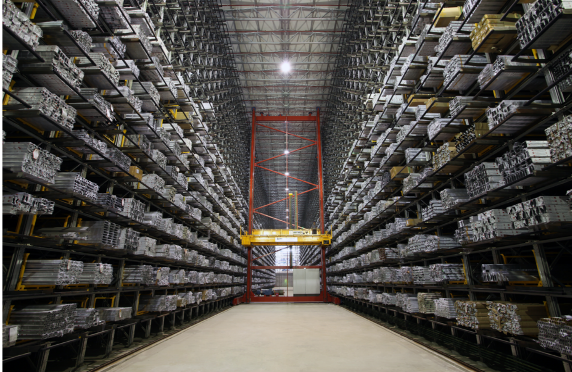
Exemplary image of the Automated Tube Storage
